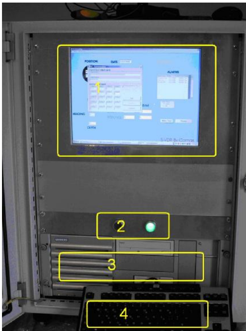
Front View of the Rack (to be changed!)
